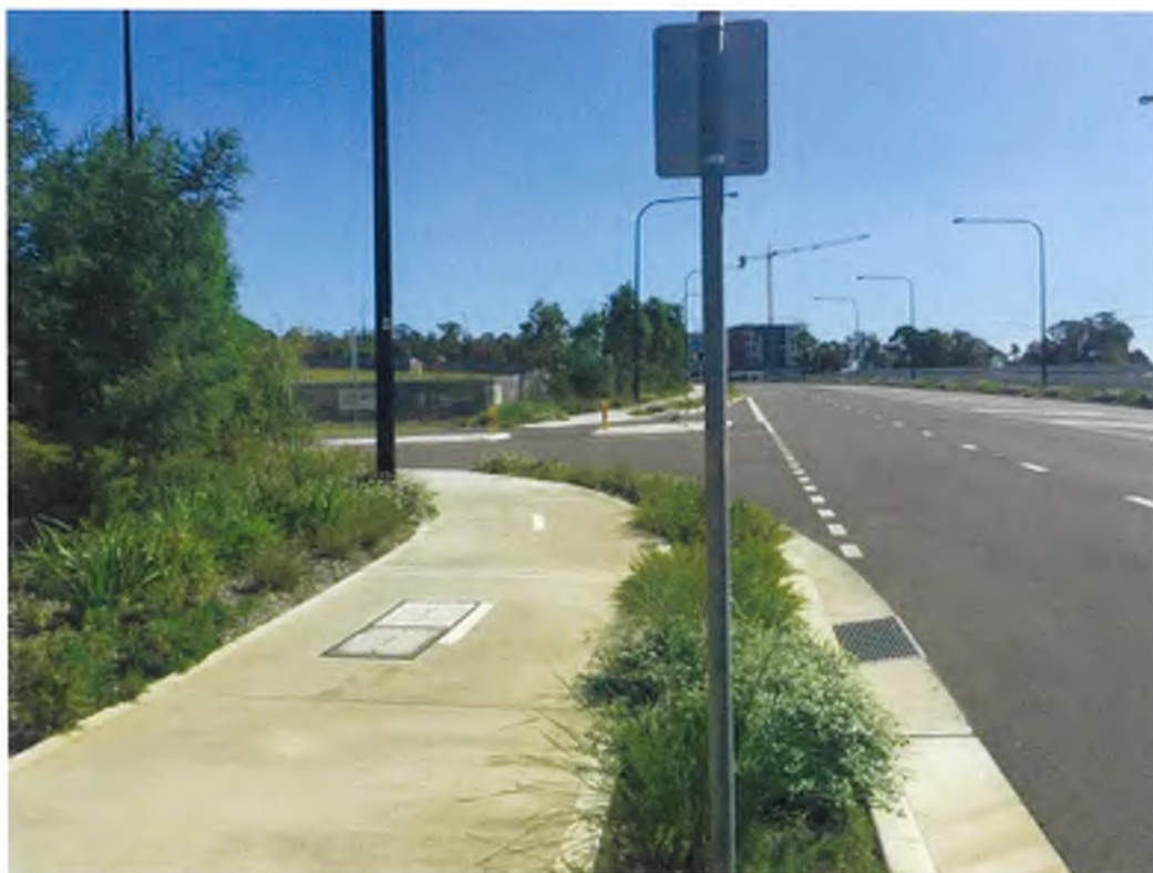
Photo 2 – Cudgegong Road / Conferta Avenue Intersection
