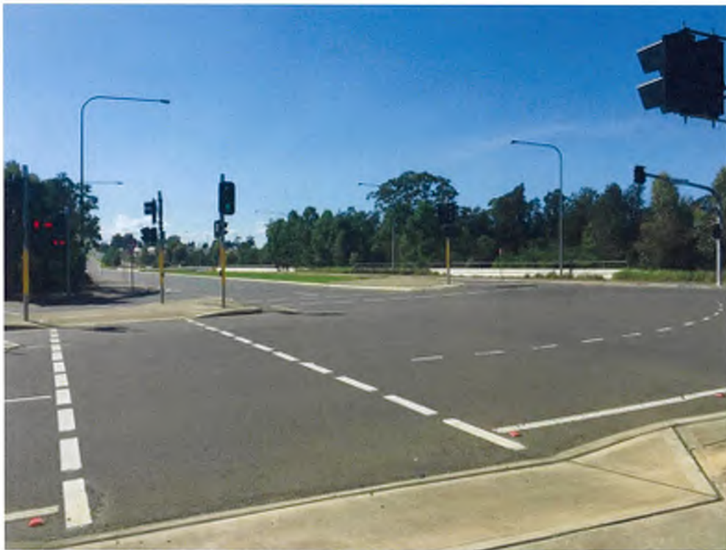
Photo 1 – Schofields Road / Cudgegong Road Intersection
